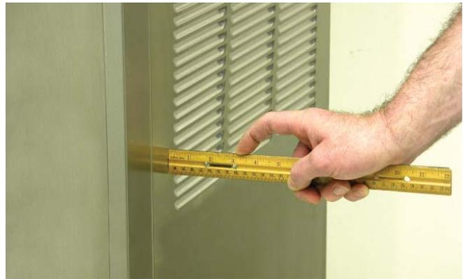
**Figure 2-1 Space and Ventilation Requirements**
